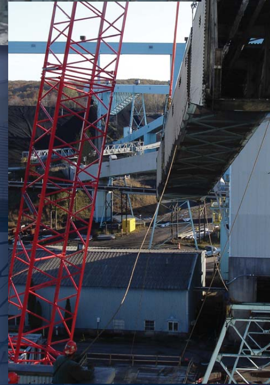
Demolition of old conveyor and chute systems
